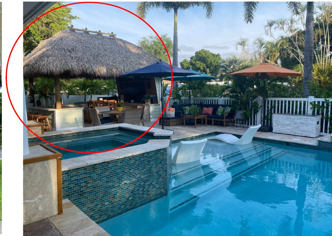
ACCESSORY SHADE STRUCTURE – FACING NORTHWEST
