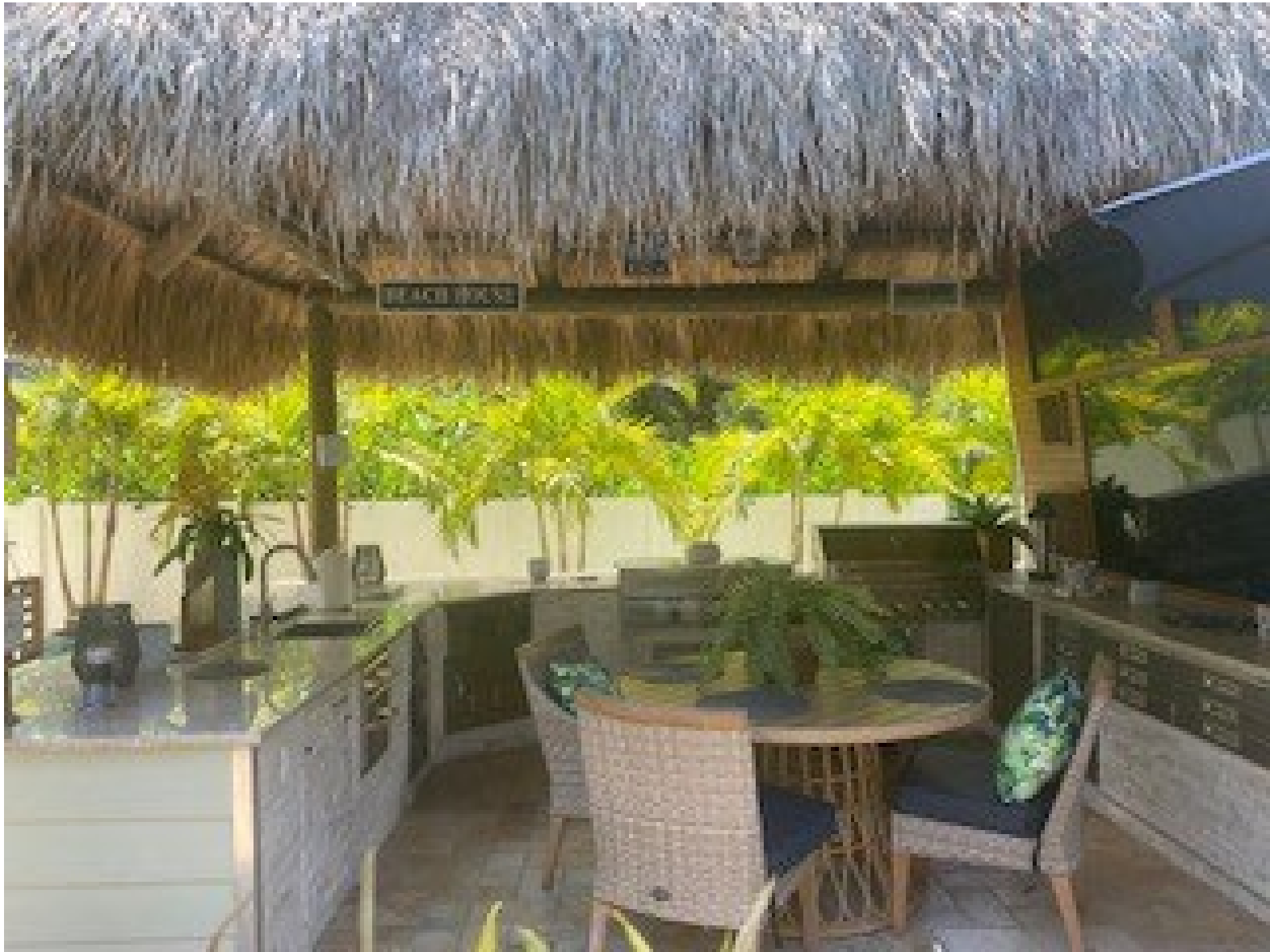
ACCESSORY SHADE STRUCTURE – FACING WEST
