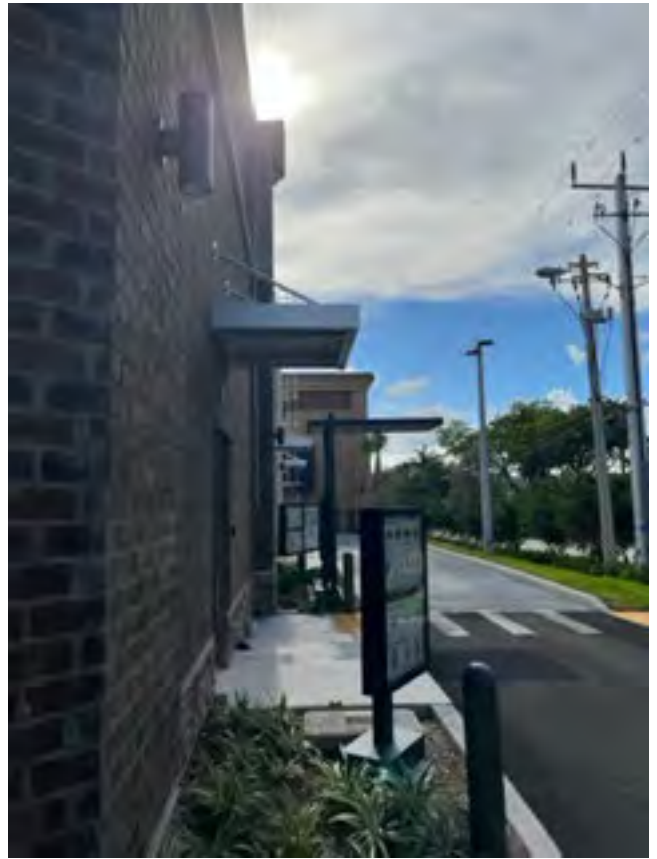
8/26/2022 This is the west side of the building
