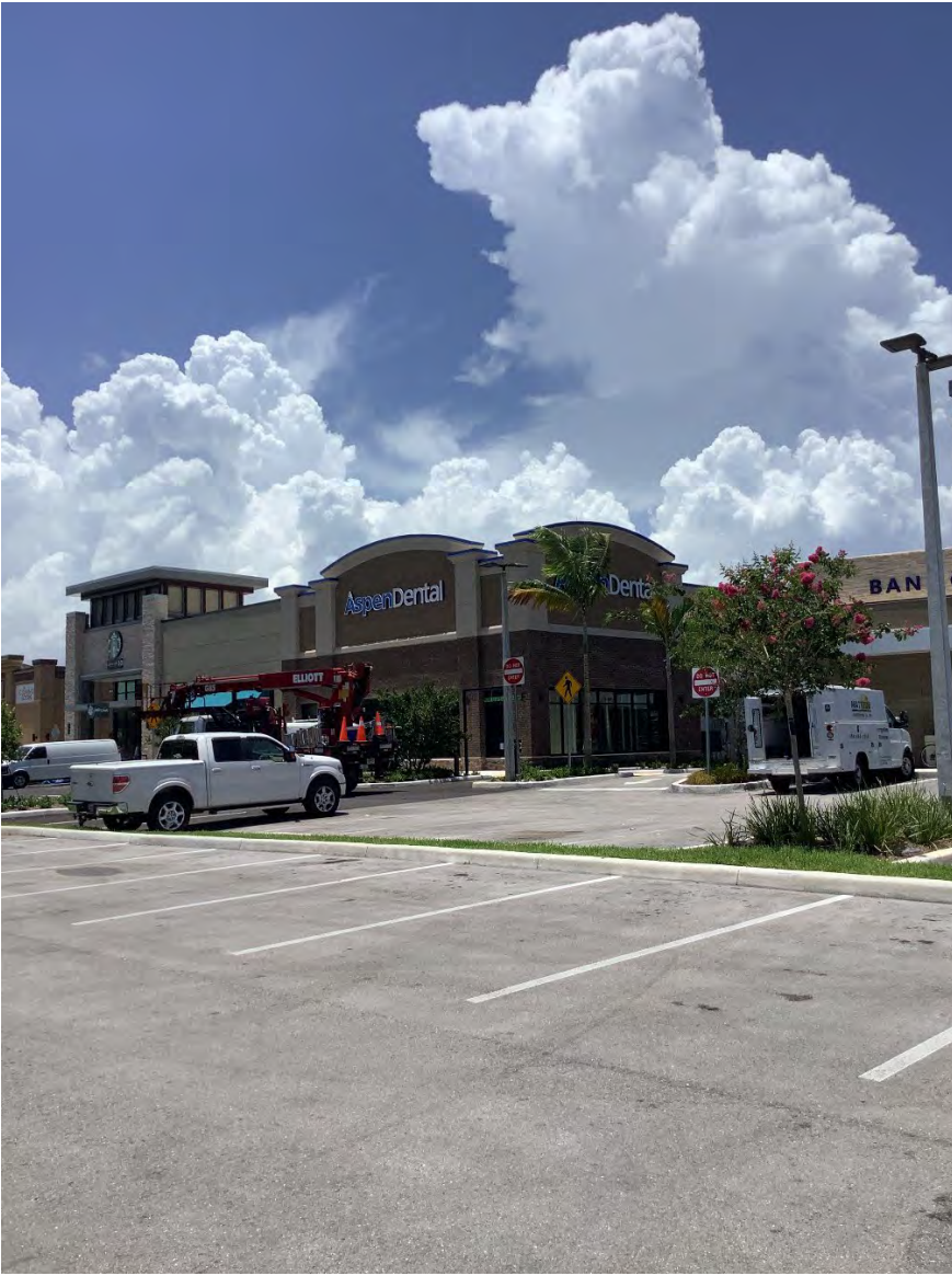
8/26/2022 Front elevation of building
