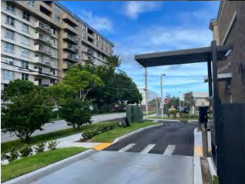
8/26/2022 facing east from the rear of the building
