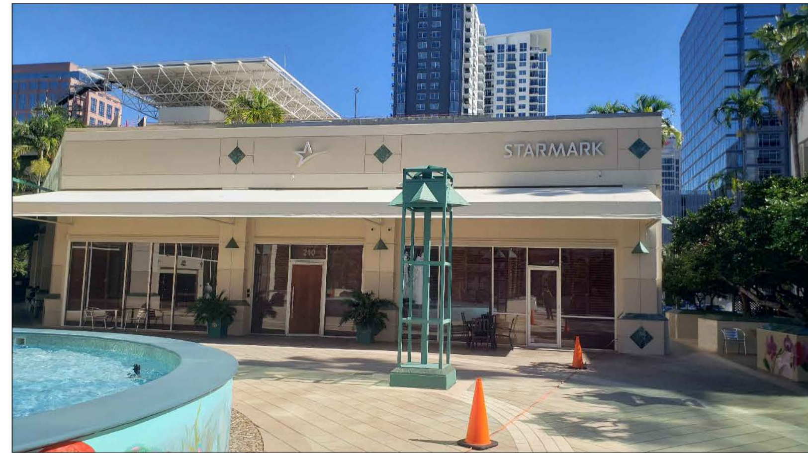
WEST FACADE OF PROJECT FACING THE COMMON PLAZA AND WATER FOUNTAIN
