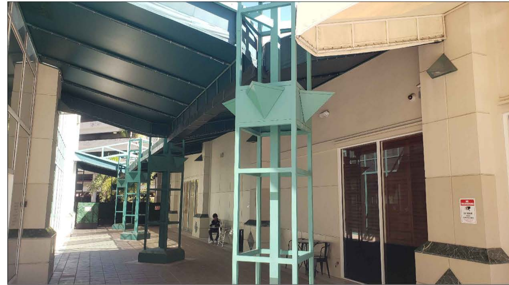
WALKWAY BETWEEN BUILDINGS ON NORTH SIDE OF PROJECT
