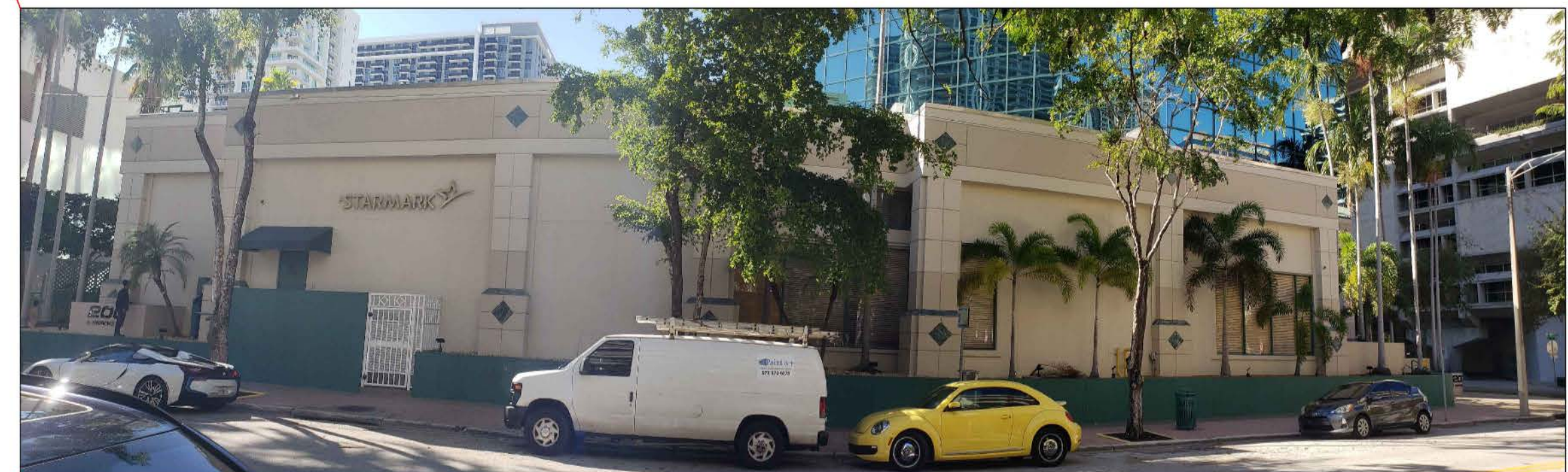
WEST FACADE ALONG SE 1st AVE
