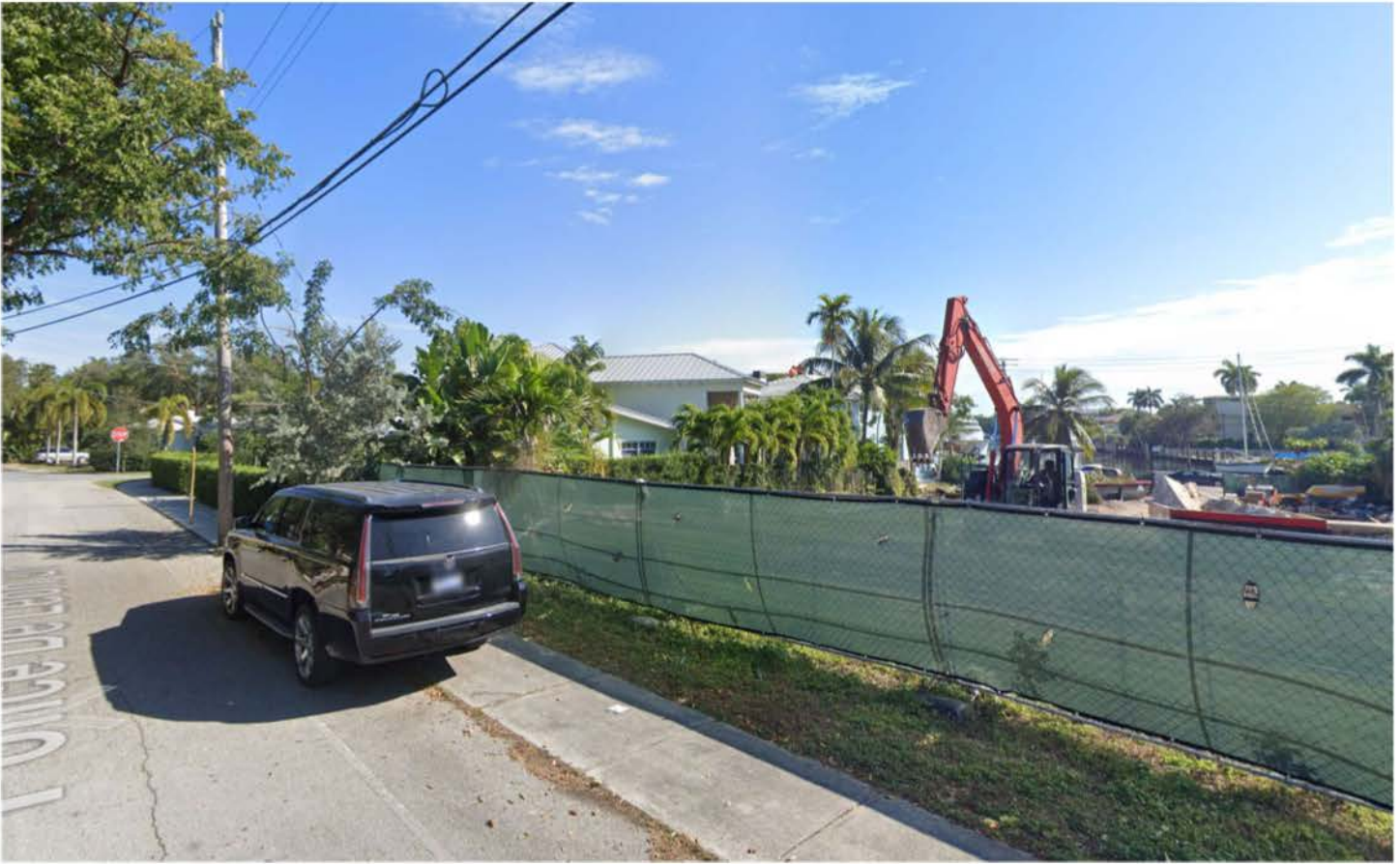
Site Photo – Facing Northeast
