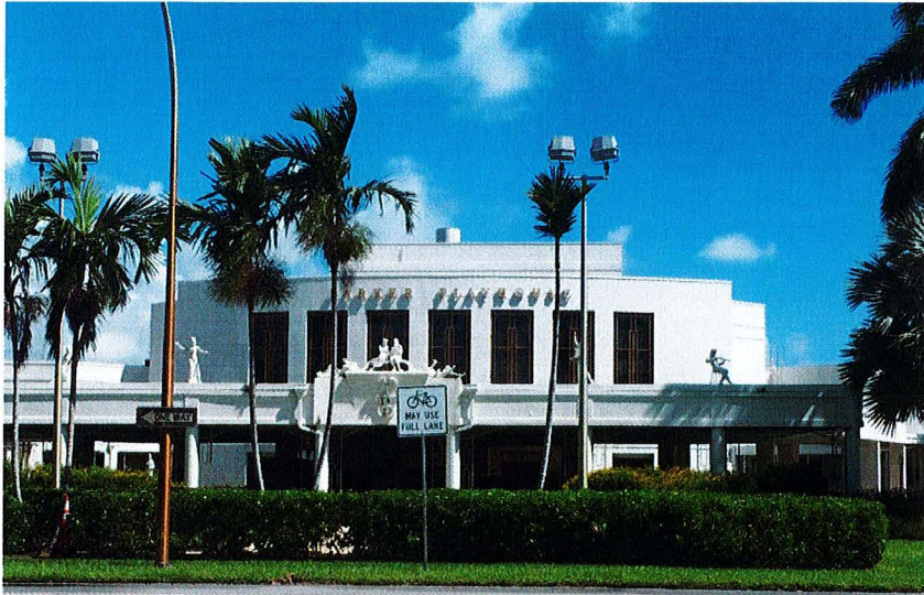
Photo Prior to Renovation (2018)
