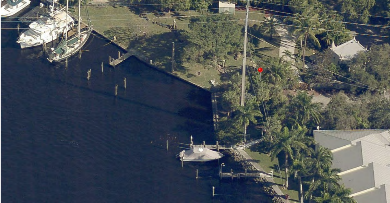
1. Southern portion of the subject site, facing north along the New River.
