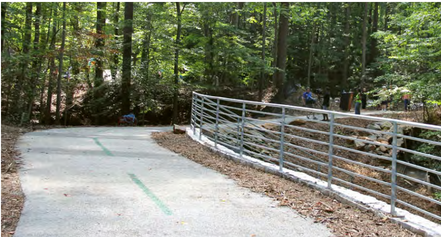
Example of a green centerline strip on a greenway trail
