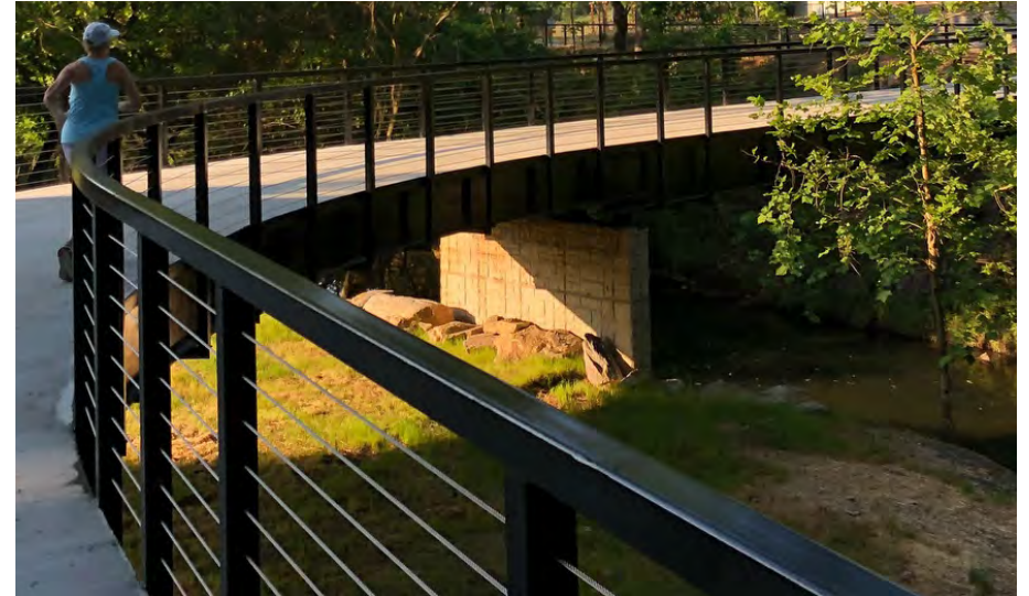
Bridges with painted finishes are timeless and suitable for urban environments
