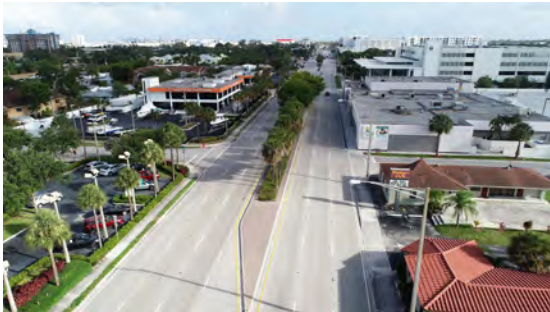
Existing condition of U.S.-1, facing south
