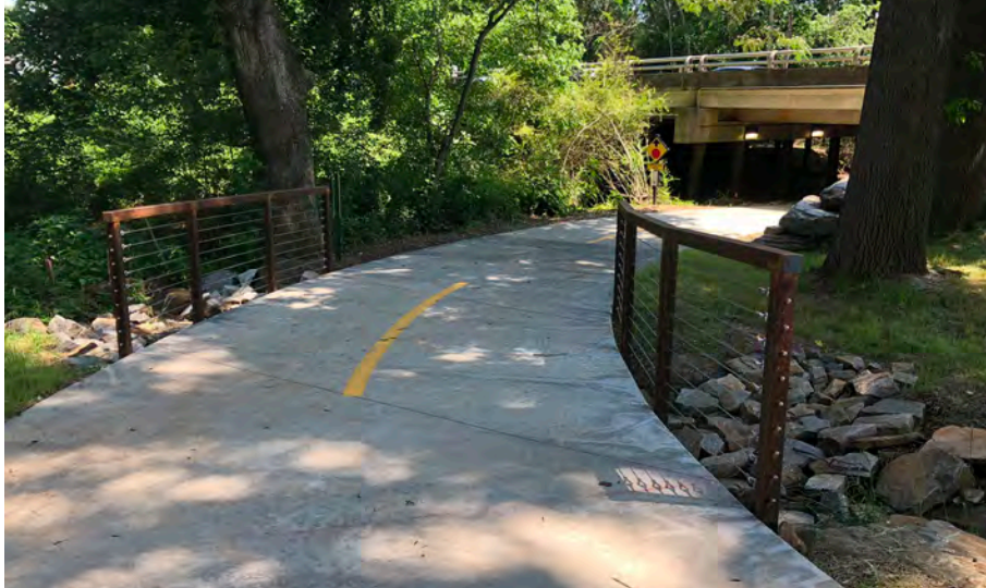
An example of the cable handrail with corten steel posts and top rail.
