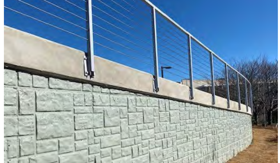
Post & Cable railing provides a safe trail edge while acting as a visually lighter option.
