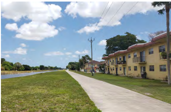
Existing conditions of the Cypress Creek Greenway Trail, looking east.
