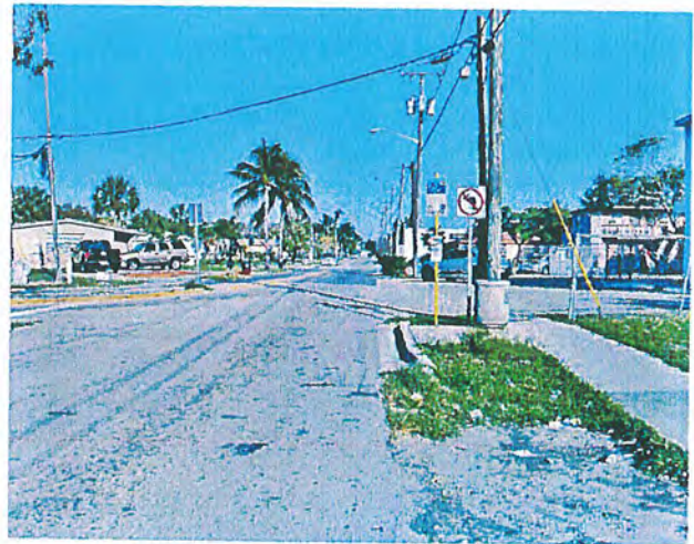
Looking North on NW 22 nd Road
