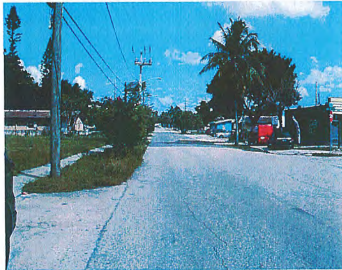
660 NW 22 Road Looking Southeast
