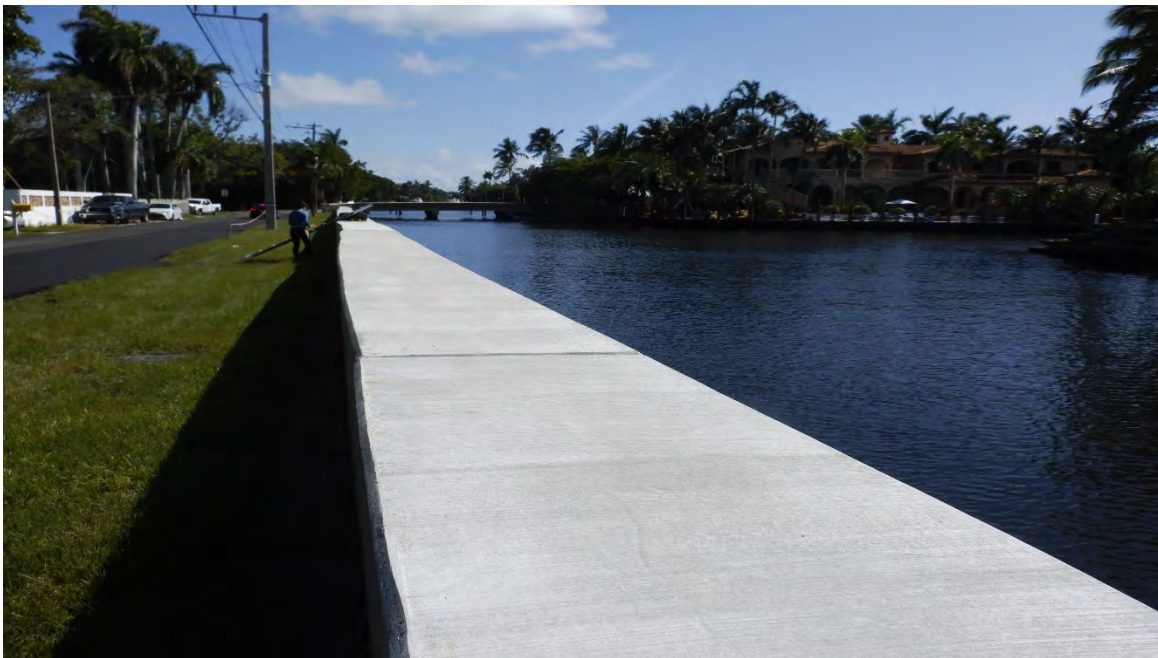
2. Southern portion of the subject site, facing north along Rio Cordova.
