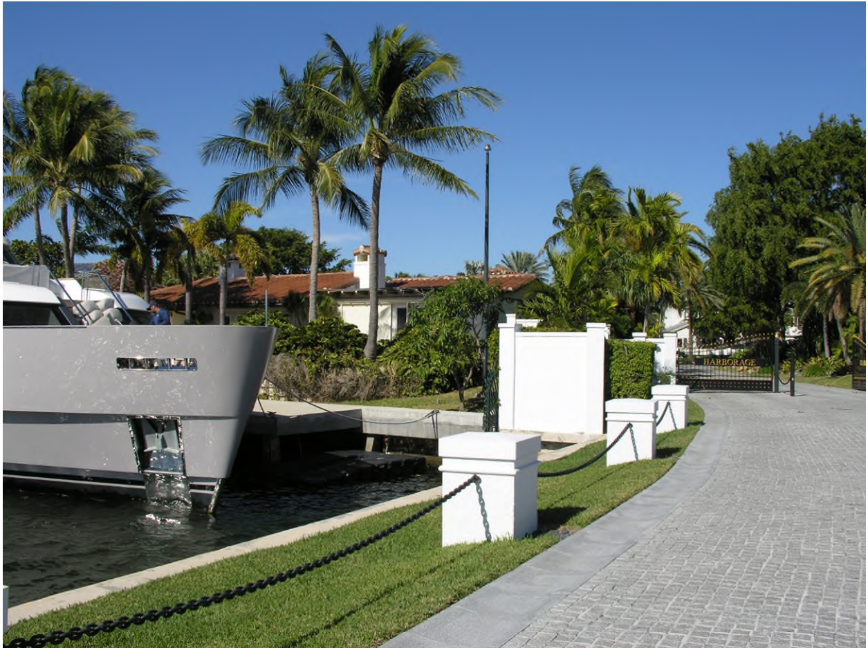
South – Rear of existing home, including gate to the east.
