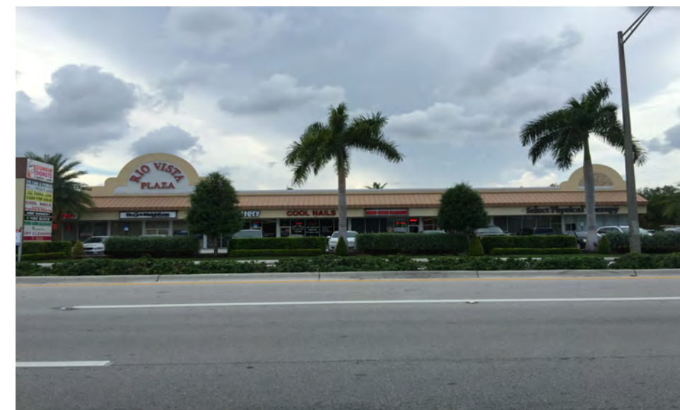
SOUTH FEDERAL HWY. LOOKING WEST
