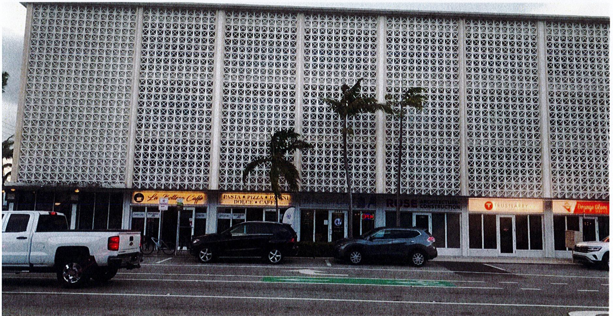
2787 East Oakland Park Building South Side of the Building
