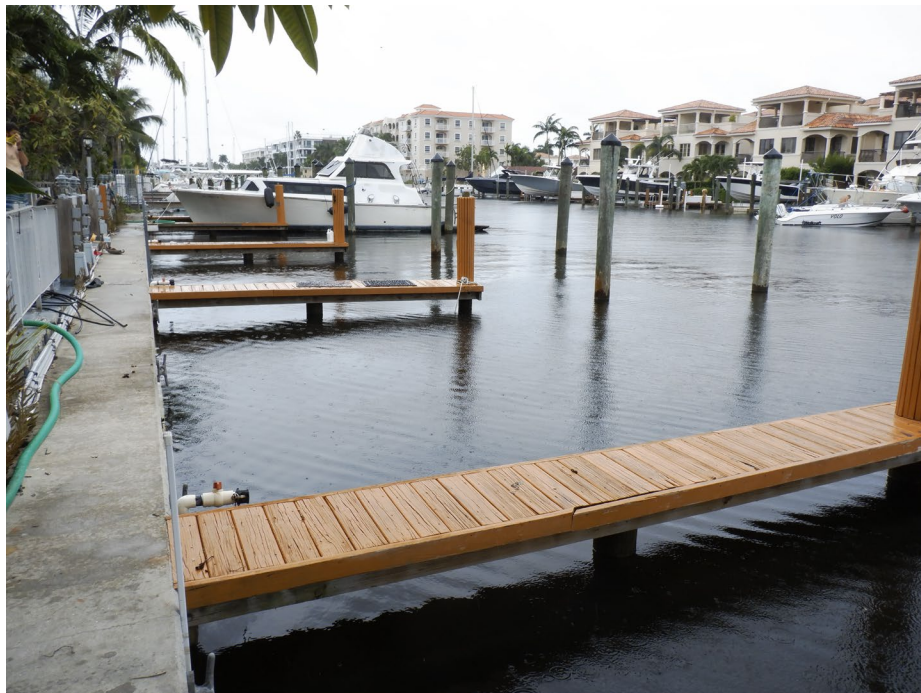
2. Northern portion of the subject site, facing south along the Rio Grande Waterway.
