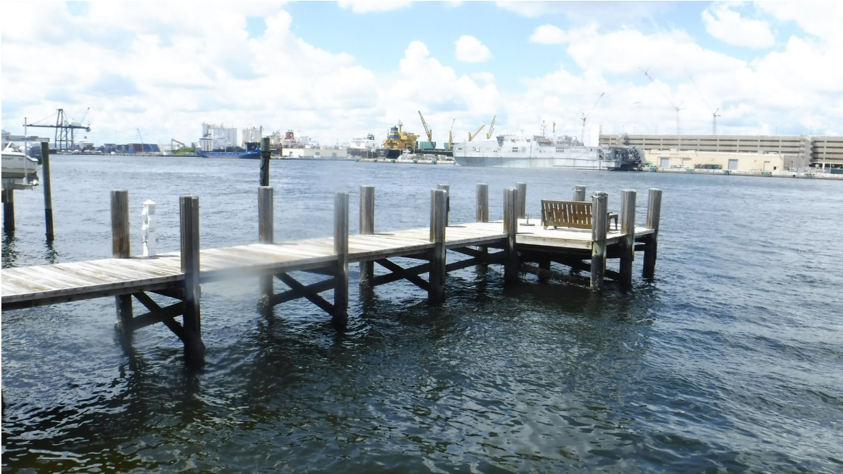
1. Northern portion of the subject site, facing southwest along the ICWW.
