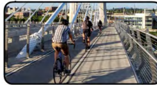
Bridge Multi-Use Paths
