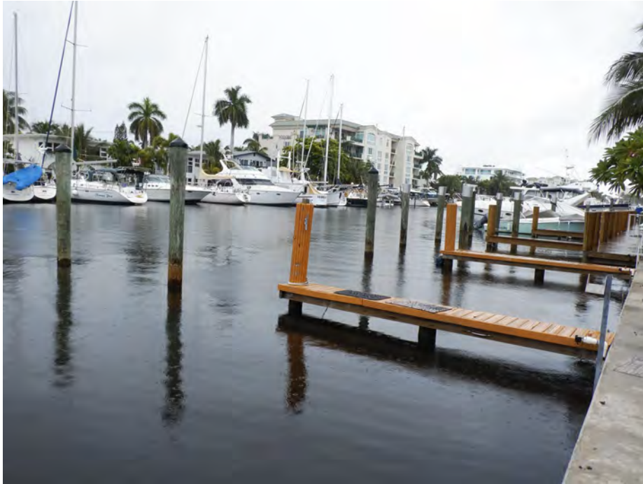
1. Southern portion of the subject site, facing north along the Rio Grande Waterway.
