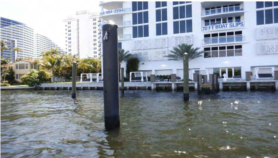
2. Central portion of the subject site, facing northeast along the ICWW.
