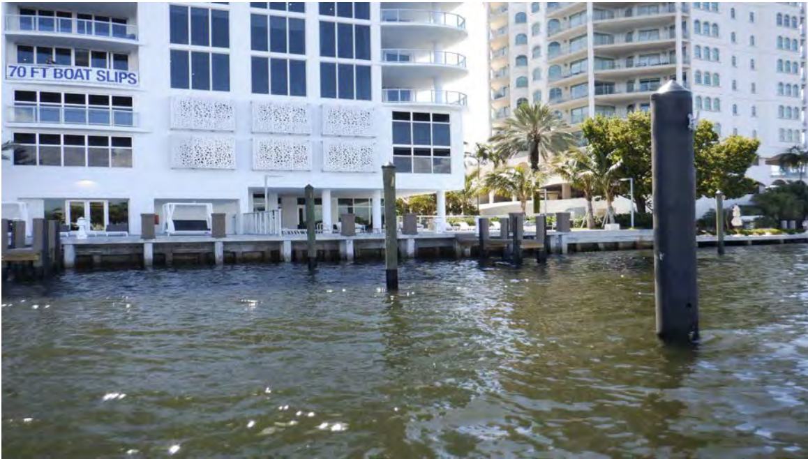
1. Central portion of the subject site, facing southeast along the ICWW.
