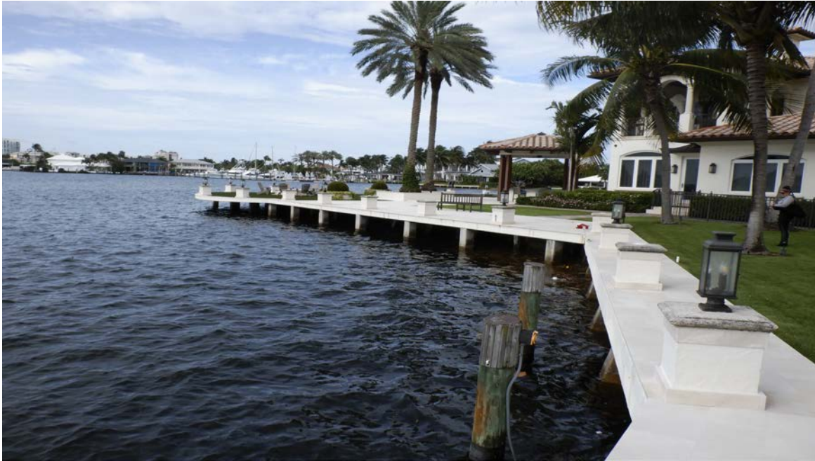
1. Northeast corner of the subject site, facing southwest.
