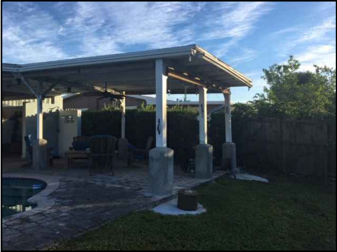
3. WEST TO PATIO ROOF
