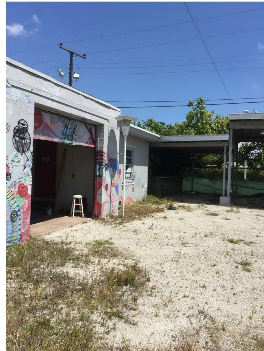
EXISTING - EAST VIEW
