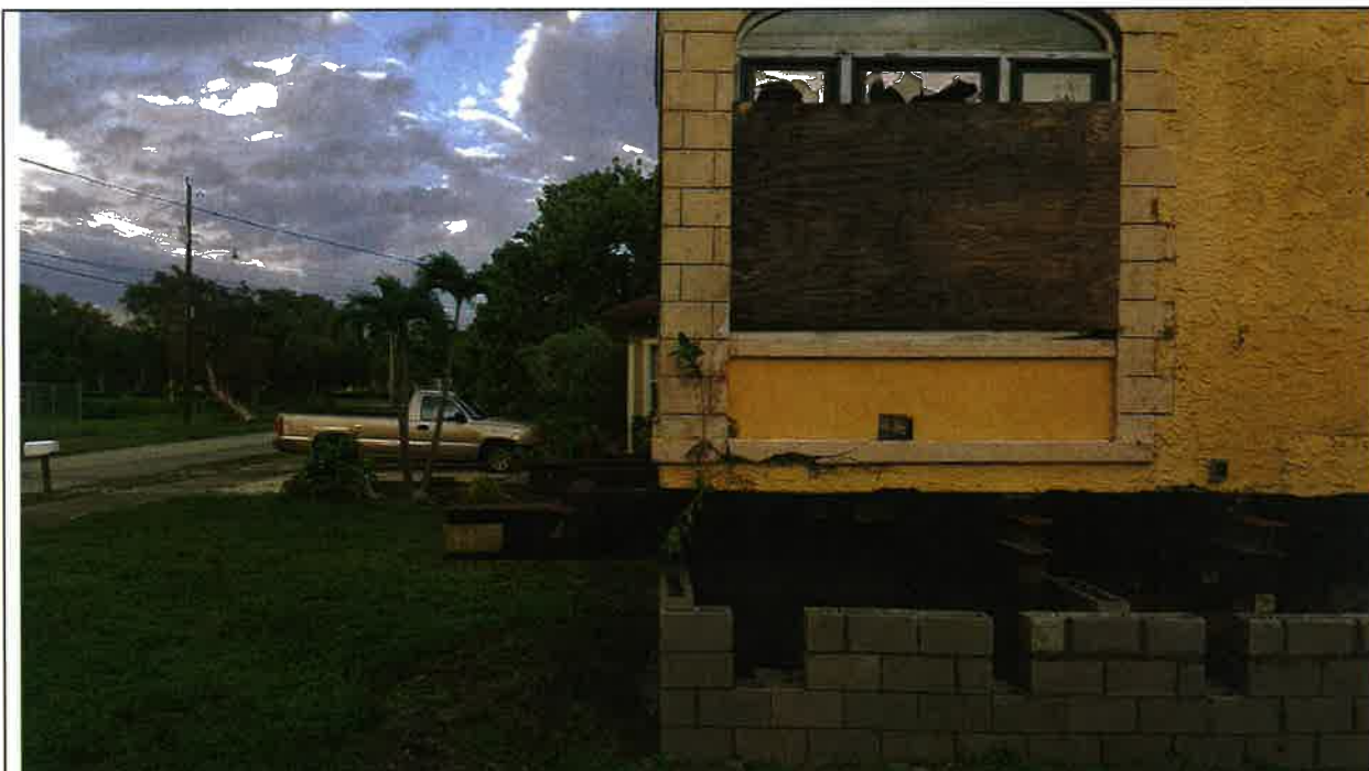
View with neighbor house 724, which is closer to property line. 9/3/2019
