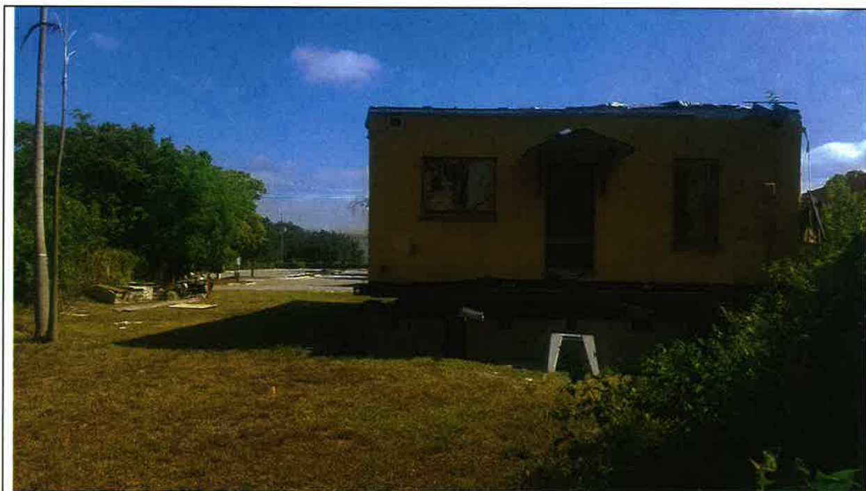
728 NW 3 Street Back/South side 8/24/19
