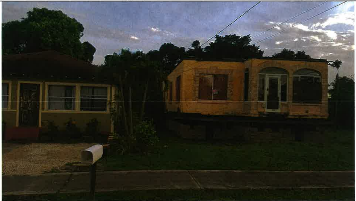
728 NW 3 Street front and east side View. 8/24/19
