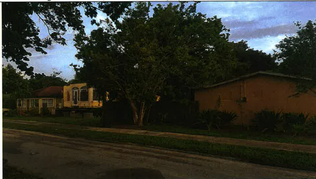
724 NW 3 ST, 728 NW 3 ST abd 216 NW 8 Ave (L to R) 9/3/2019
