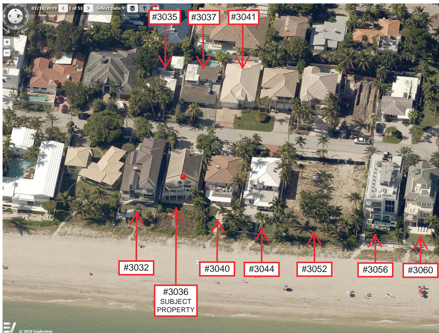
BCPA AERIAL DATED 1/14/19 - EAST ELEVATIONS - LOOKING WEST
