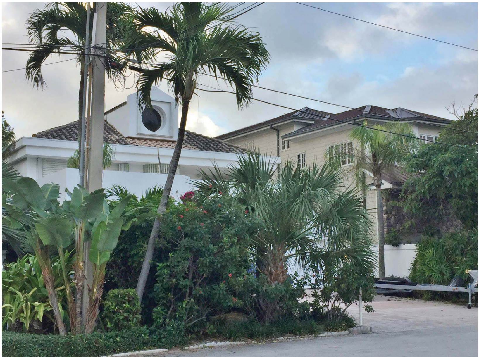
#3036 (SUBJECT PROPERTY) FRONT (WEST) ELEVATION ON THE LEFT WITH #3032 NEIGHBOR ON THE RIGHT
