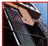
PERFORATED METAL GUARDRAILS
