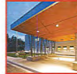
WOOD PANEL SOFFIT ACCENTS
