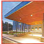
WOOD PANEL SOFFIT ACCENTS
