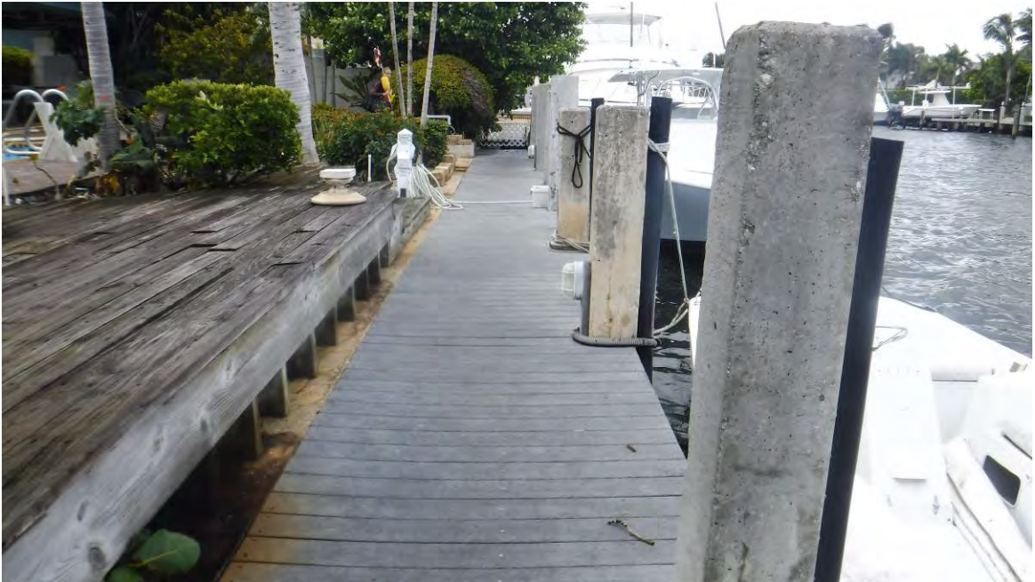
2. East portion of the subject site, facing west.
