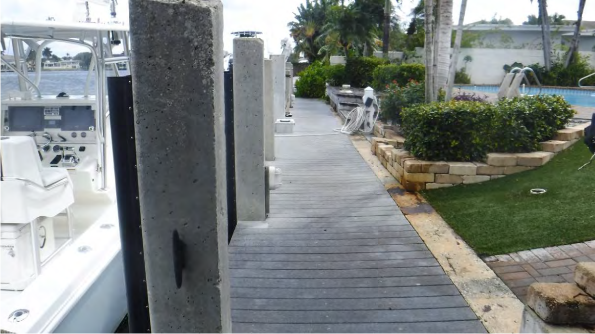
1. West corner of the subject site, facing east.
