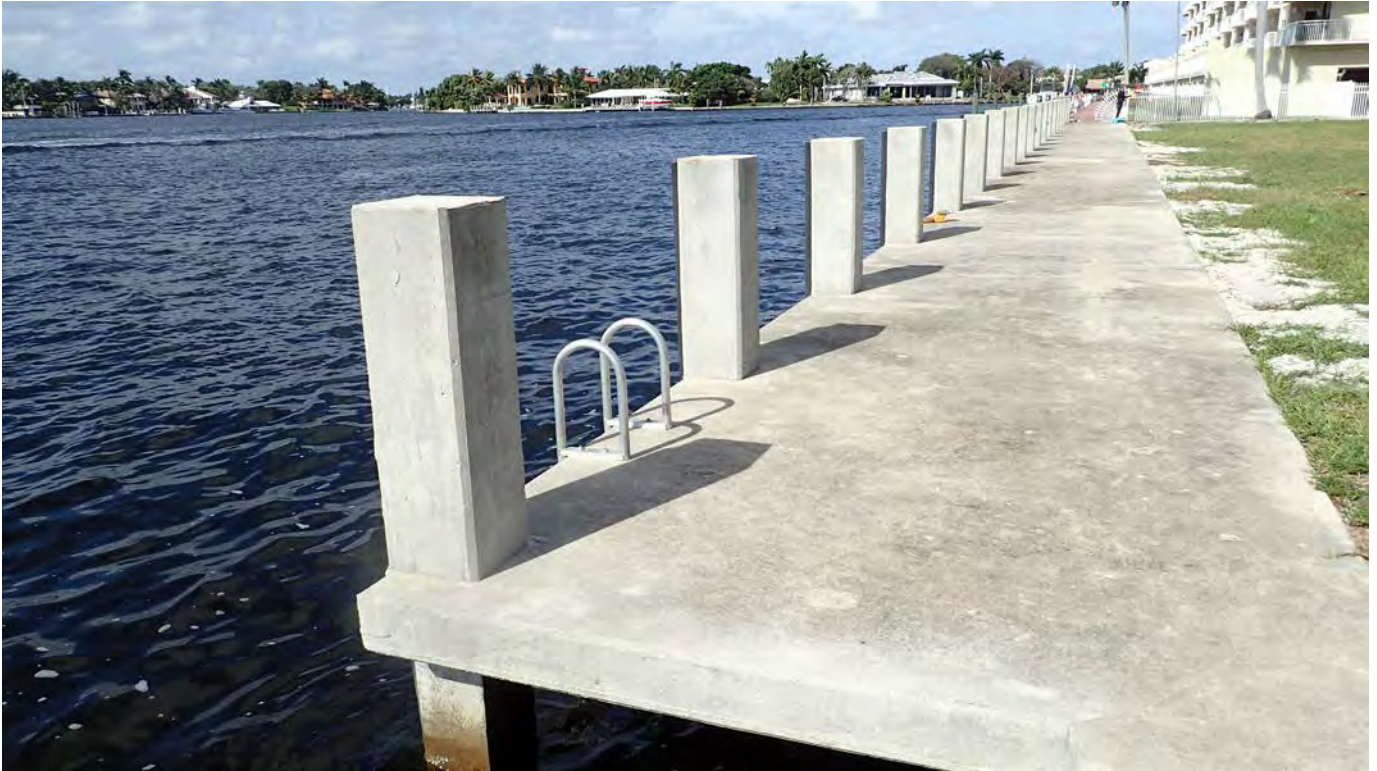
1. Southeast corner of the subject site, facing northwest.
