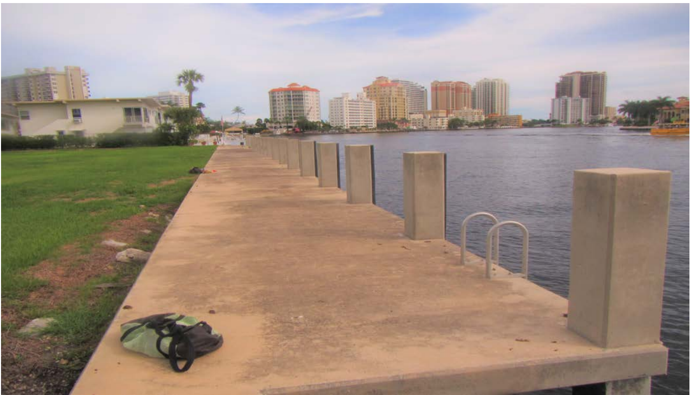
2. Northwest corner of the subject site, facing southeast.
