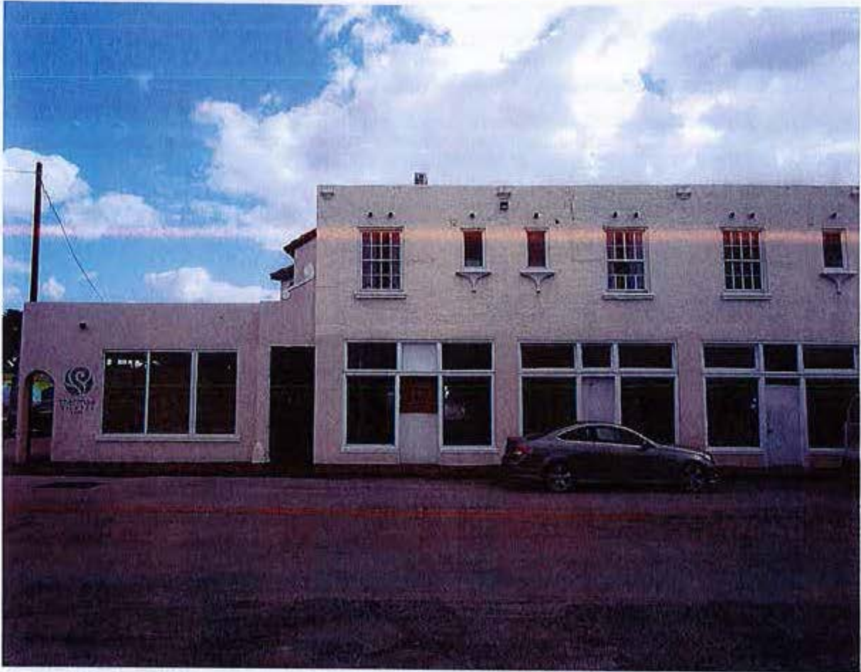
Bays along NE 9 th Street in Progresso Plaza where Patio Pizzeria will be located.
