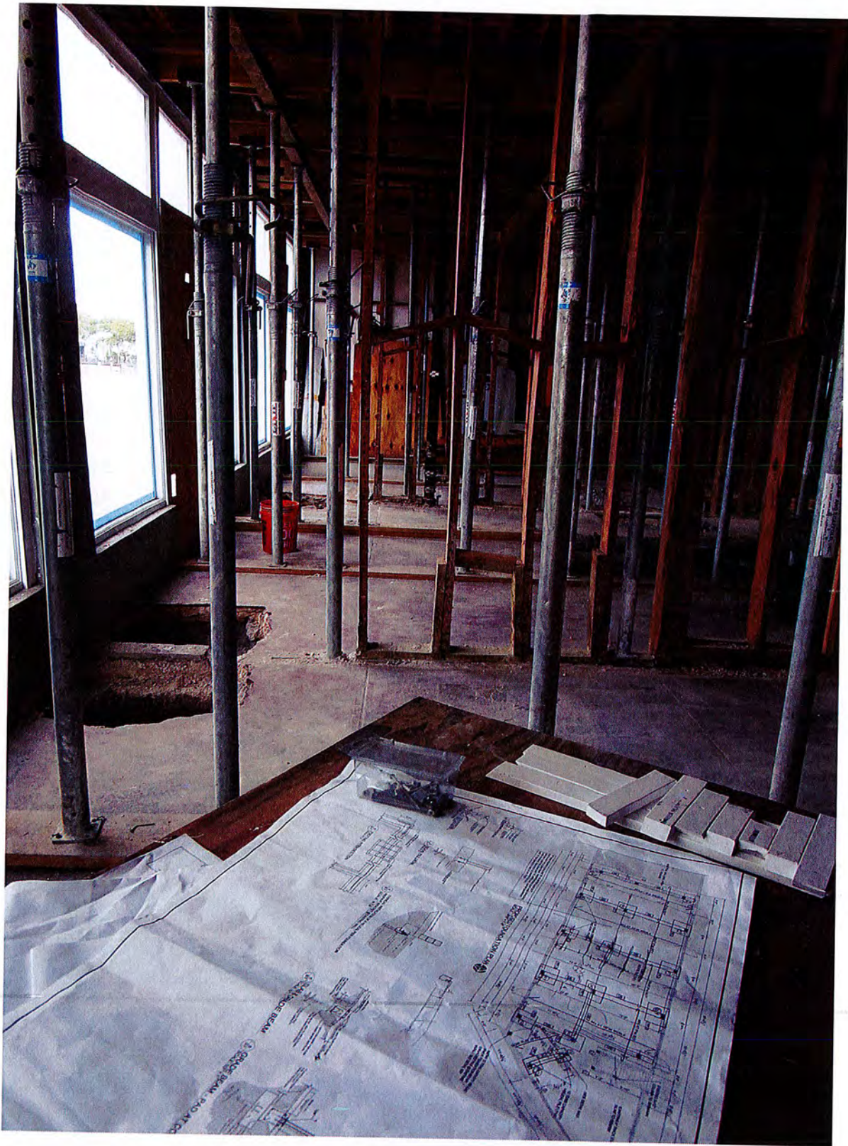
Bays Requiring Total Reconstruction for Bar-Restaurant Re-use.
