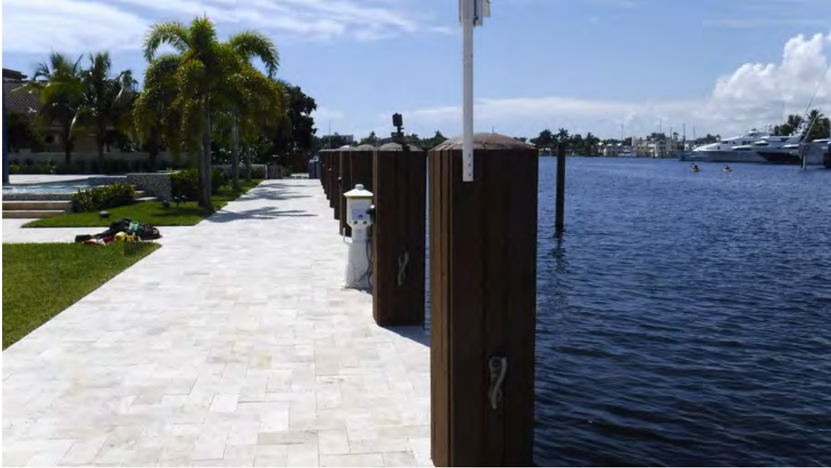
1. North corner of the subject site, facing south. Note existing concrete dock.
