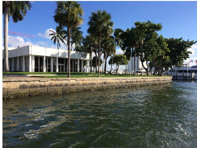
Figure 2.8.2 Seawall No. 19 Supports Parking and Structure Facilities
