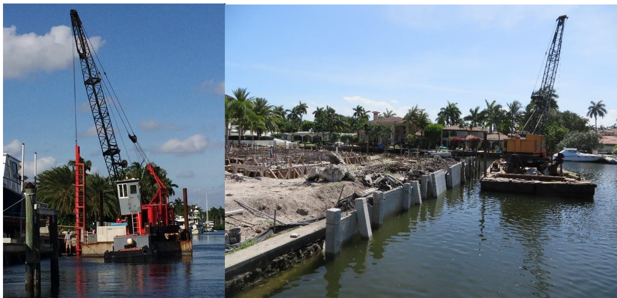
Figure 4.10.1 Conventional Seawall Installations
